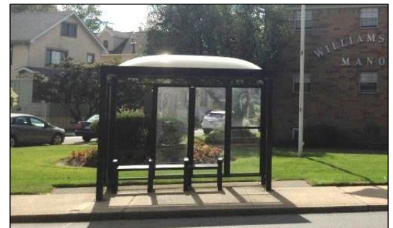
Bus shelter along Liberty Street
