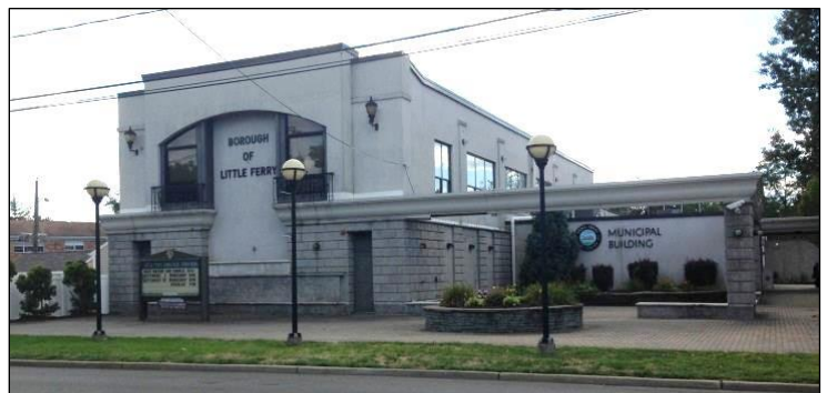
Little Ferry Municipal Building
