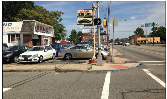
Poor sidewalks along Route 46
