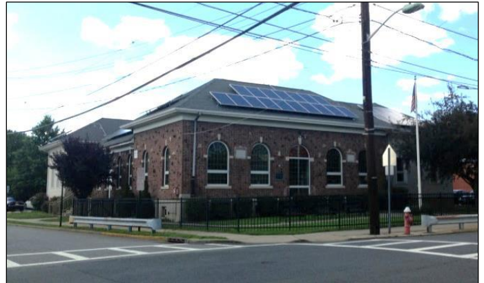
Public Library with roof-top solar panels
